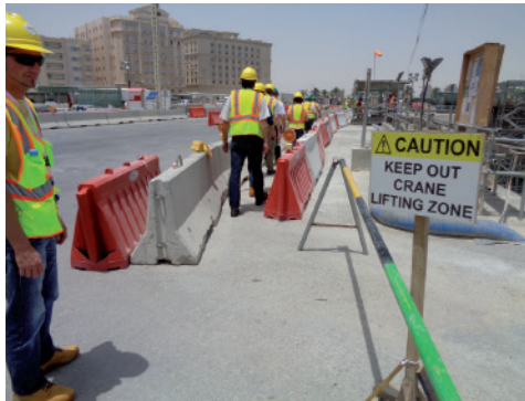
Technical protective measures: separation between vehicle traffic and pedestrians.
