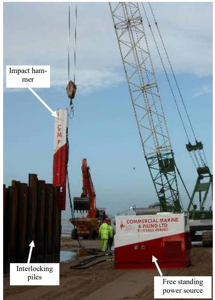
Free riding impact hammer driving interlocking piles following a vibrator
